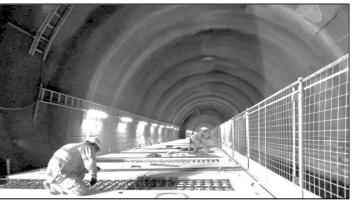
A major milestone in the construction of the new Crossrail station at Liverpool Street has been reached with the completion of the two new platforms over 30 metres below ground. The two 240-metre-long platforms, constructed as part of the Crossrail programme, were pre-fabricated in more than 500 pieces at a state-of-the-art factory over 130 miles away near Sheffield. They were then transported to London, lowered down the station's main shaft and pieced together.
